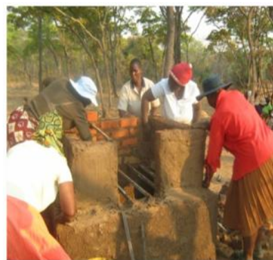
Construction of the clay oven. Photo courtesy of Taurai Matope
