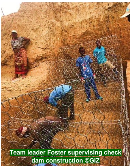
Check-dam construction in progress ©GIZ
