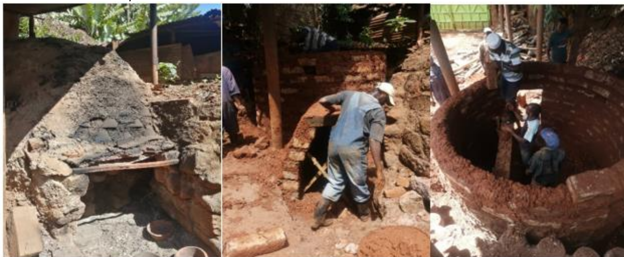
Support for construction of Kiln for curing ICS for Female producer in Kiambu County
