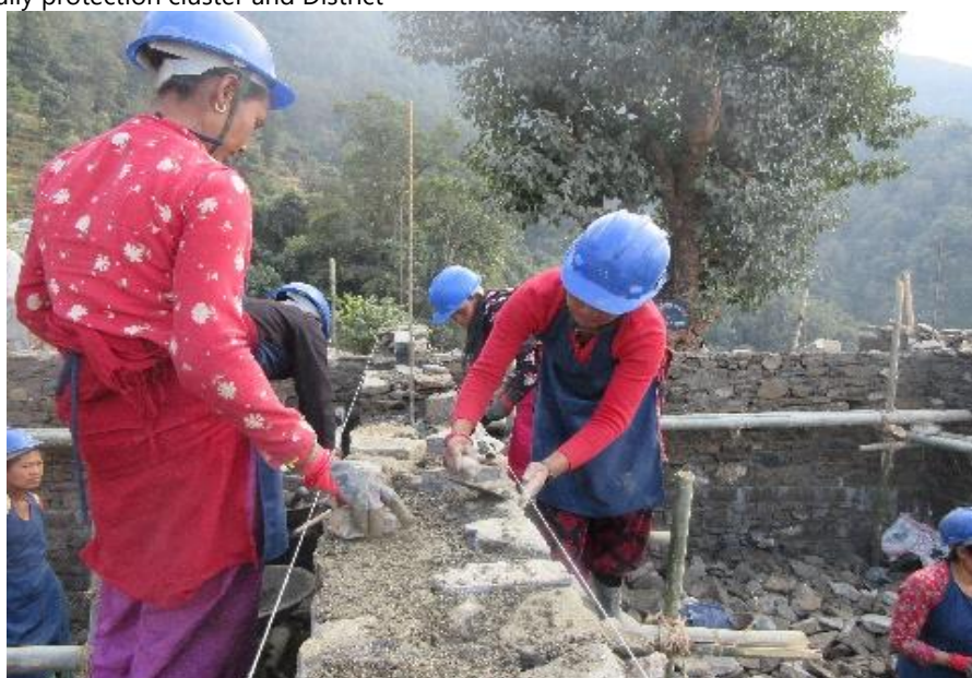
Women trained in masons working to construct their cooperative building
