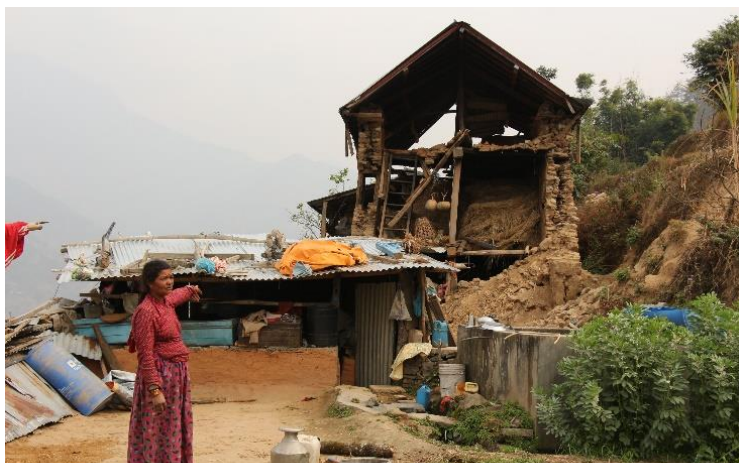
A woman showing her house damaged by earthquake
